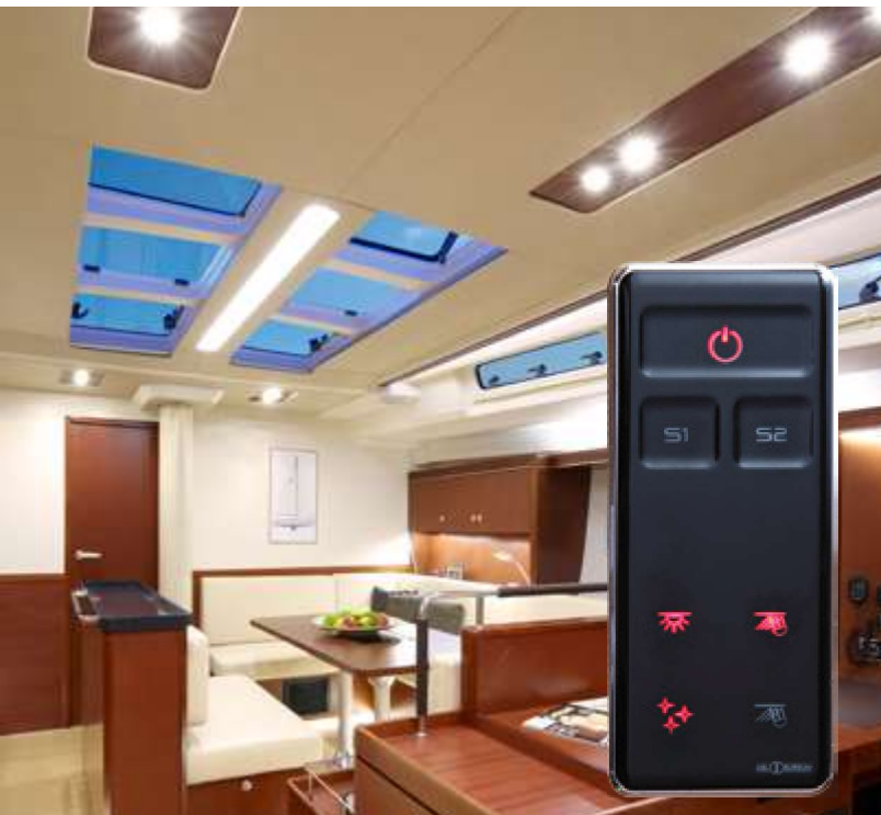
5 SLS - Intelligent Smart Lighting System. Touch screen controller & dimmer.
